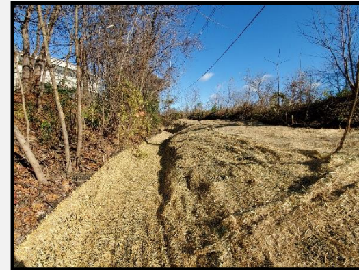
South Fourth Street Storm Sewer System Maintenance
